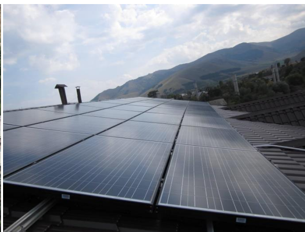
Figure 8. Grid-connected 17 kW Solar PV station at the roof of YMCA/Spitak building (2015)
