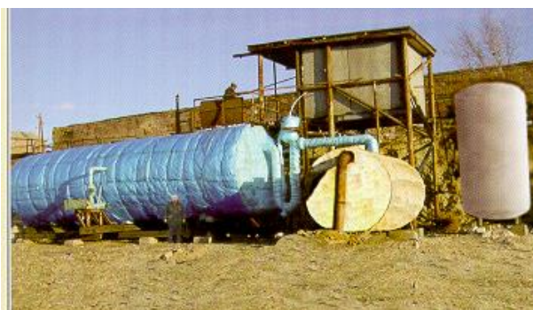
Figure 14. Biogas plant in Bartsrashen, Armenia (bioreactor 52m2)
